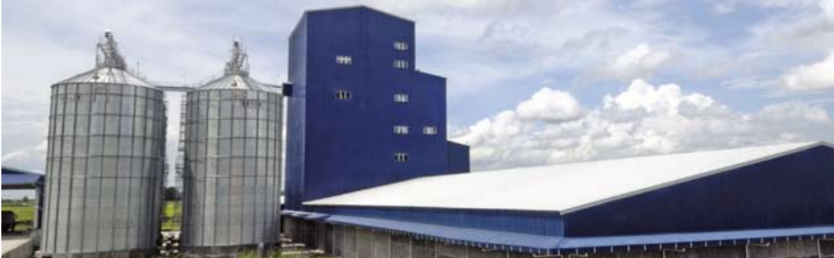
Feedmill plant in The Philippines, 40 t/h. Process : post-grinding. Engineering by customer and Stolz.
