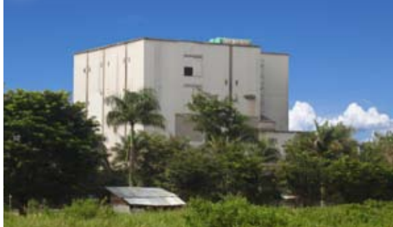
Feedmill plant in Indonesia, Grinding, mixing, and pelleting lines by Stolz.
