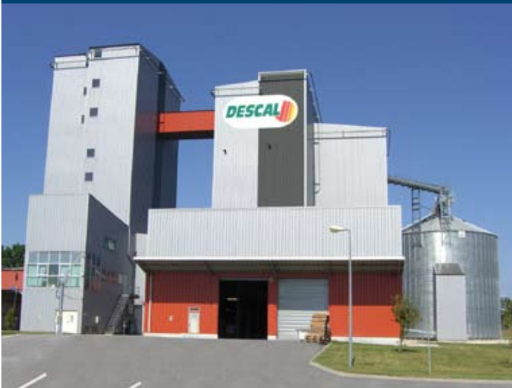
Feedmill plant in Agen (France), 40 t/h. Process : post-grinding. Engineering by Stolz.
