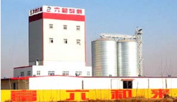
Feedmill plant in Shandong (PR China). 100% of equipment by Stolz. Engineering : local.
